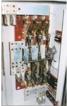
Double Pole, Double Throw 4000 Amp Switch
