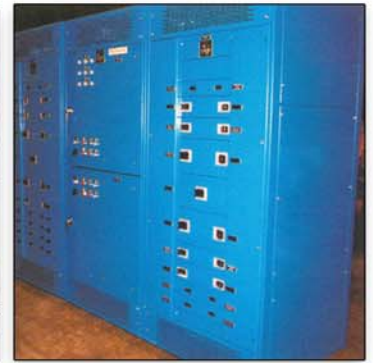
Low Voltage Metal-Enclosed Switchgear
